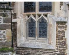
The cementitious render to the base of part of the South Chancel wall is in poor condition in parts and should be removed and the underlying stonework made good.
