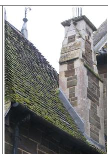
There is significant moss growth to the northern faces of the main roofs and to the vestry roof. This should be brushed clear during a period of dry weather.
