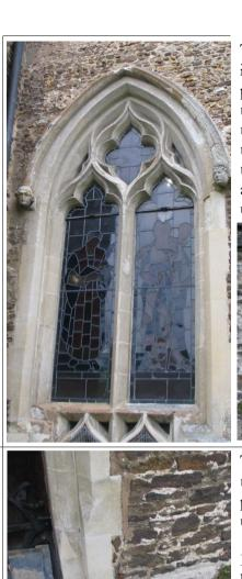
The stonework to window W3 is in a poor state in parts. The hood mould appears to have had previous render repairs which are either themselves failing or as discovered recently on the East window the render is merely masking the state of decay of the stone behind, and is the highest priority. The stone to the lower rail and jambs is in need of attention but less urgent.
