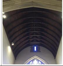
Internally the Nave, North aisle and Chancel ceilings all appear in good condition, though being dark stained and in the shadow a closer inspection is recommended when opportunity allows.
