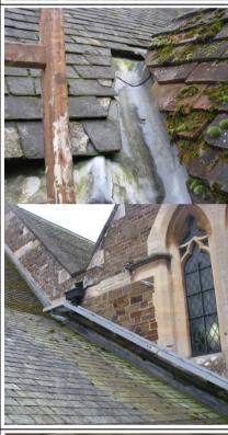
Access to the roofs and particularly the upper 'hidden' valley between the Nave and North Aisle is awkward. Whilst from the point of view of security this is a good thing, access for maintenance other than during dry periods is impractical and unacceptable by modern health and safety standards.
